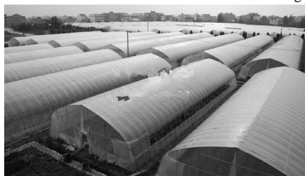
Group Arrangement of Greenhouse
